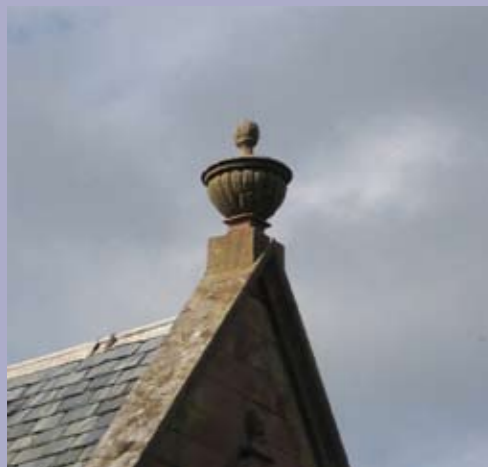
A stone terminal on a gable end
