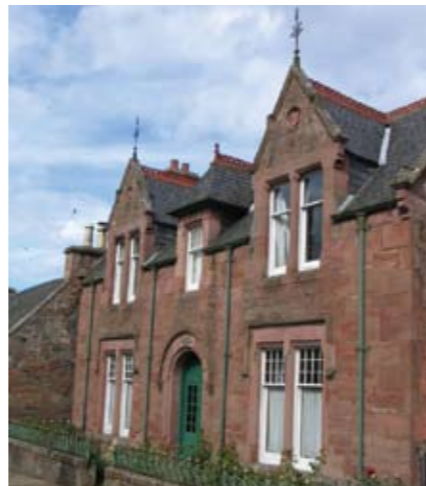
Cast iron finials were frequently complemented by cast iron railings cresting and rainwater goods
