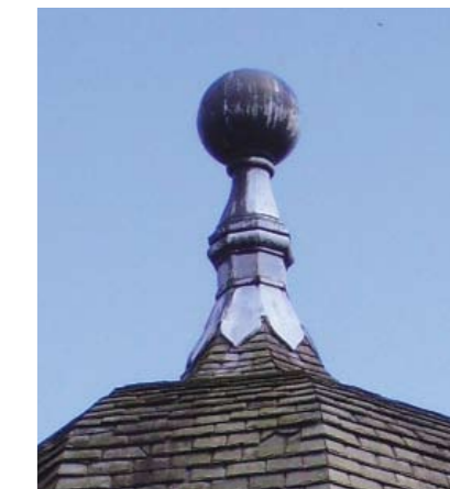
A lead concealed finial
