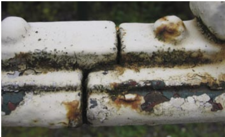
Image: Traditional cast iron joints owe much to woodworking principles © D S Mitchell
