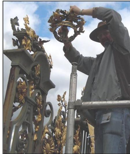
Simon Doyle removes one of the crowns with failing fixings.
